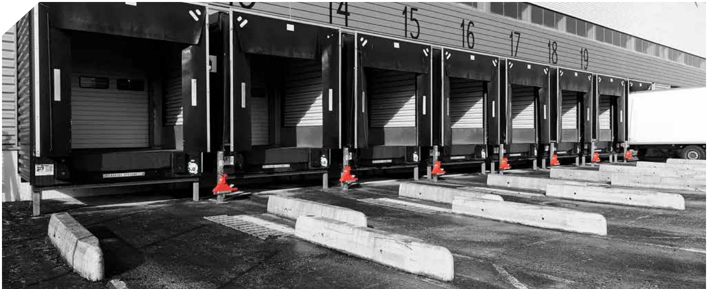
ID Logistics Châtres securing its docks with the POWERCHOCK restraining system.
